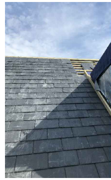
SIGA 32 Blue Grey Natural Slate (5mm) - National Parks approved (as installed on a recently completed conservation project in Hexham)
