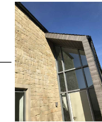
TRESPA CLADDING NATURAL MYSTIC CEDAR [PU 22] and TYNE VALLEY RANDOM STONE and uPVC Black Rainwater goods collectively shown as installed on a recently completed project
