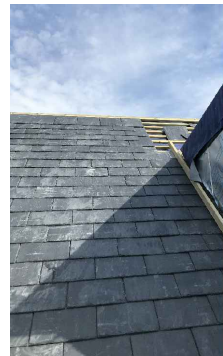
SIGA 32 Blue Grey Natural Slate (5mm) - National Parks approved (as installed on a recently completed conservation project in Hexham)
