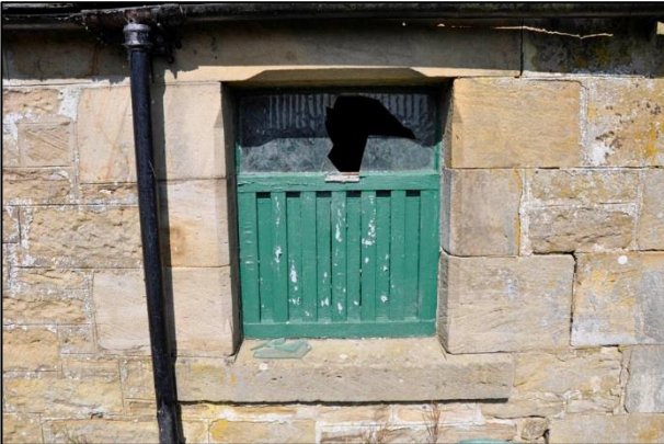
Figure 21: Detail of stables opening with chamfered stone surround
