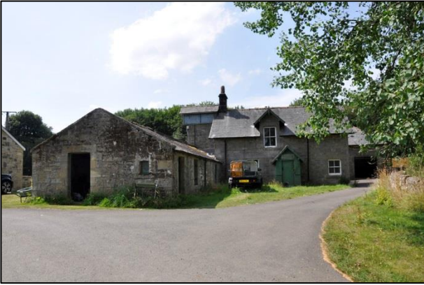
Figure 17: Evistones Cottage and stables. Cart shed/vehicular opening to hay barn at rear
