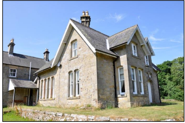
Figure 11: Evistones House with former staff quarters range to the rear
