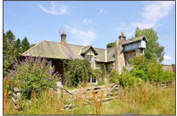
Figure 18: Cottage with dormer window and water tower with tank, c.1900
