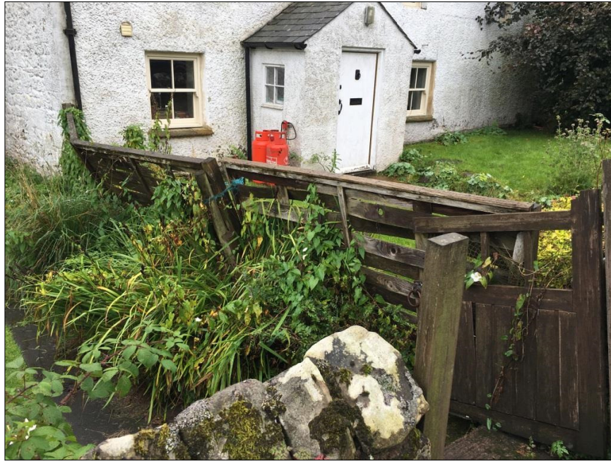
As referred to above, the boundary fence and pedestrian access gate
