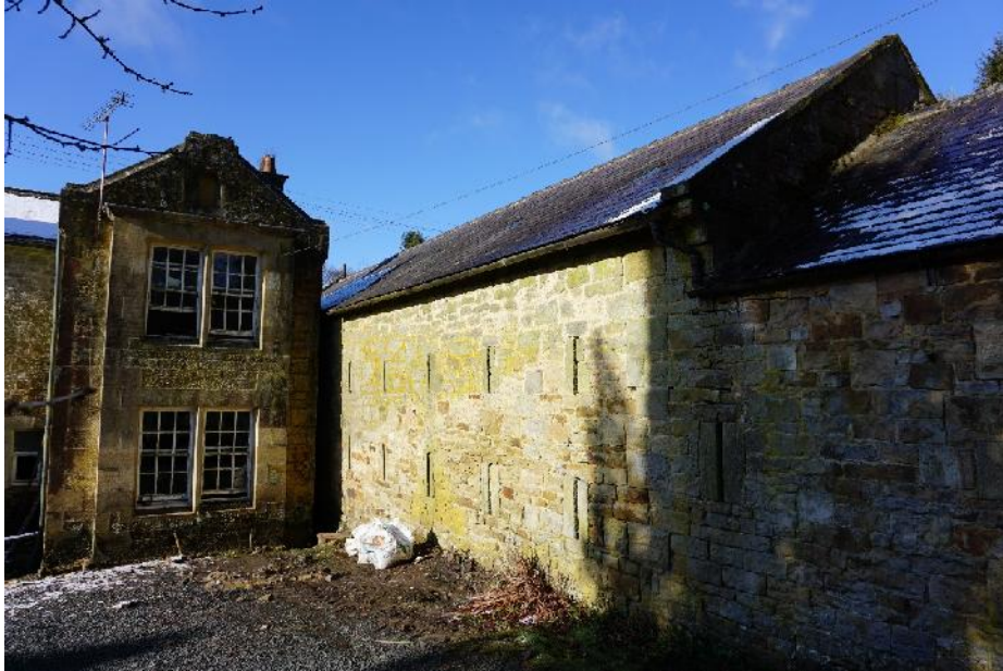
PHOTO 1 – Southeast Elevation (facing west)
