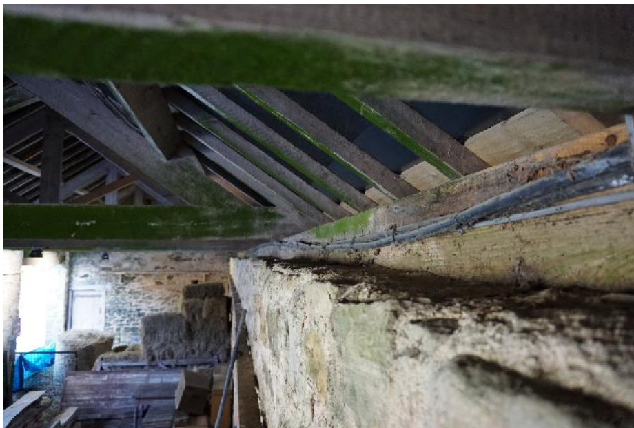
PHOTO 4 – Eaves Detail (300x150 timber wallplate)
