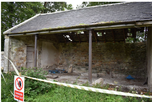
Main section of building with open colonnaded front
