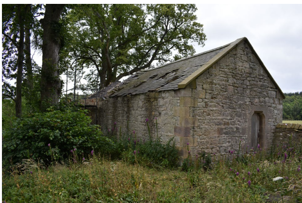
Rear and gable of main section of building
