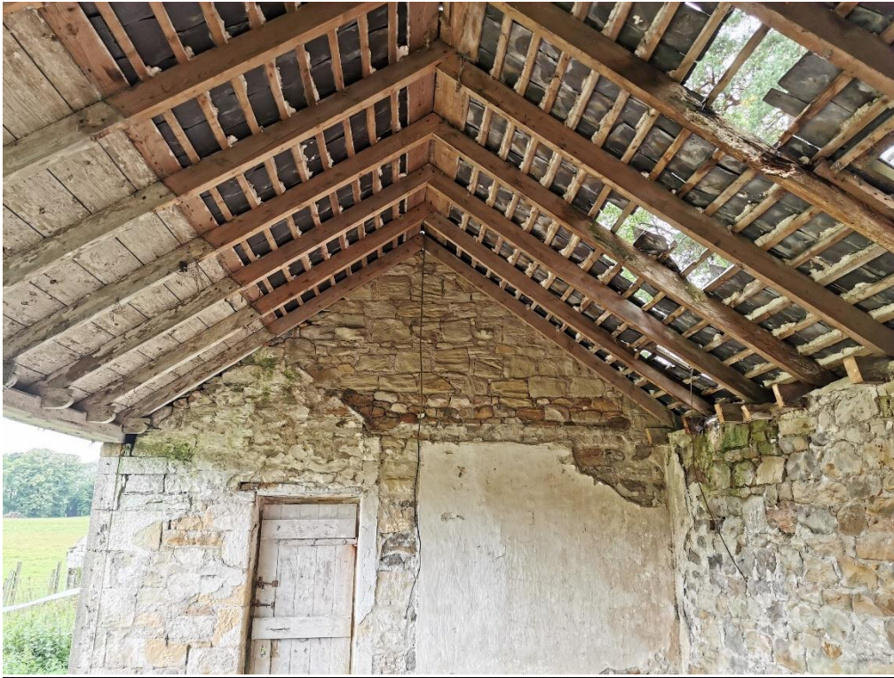
Photograph No. 3 – internal view of roof structure
