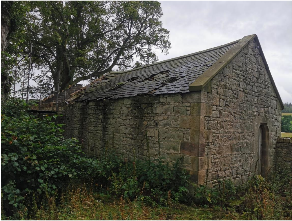
Photograph No. 5 – view from rear of building
