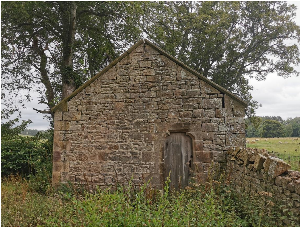
Photograph No. 4 – northwest gable
