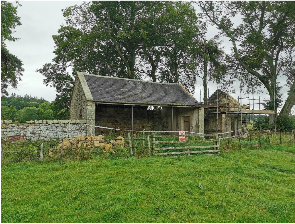
Photograph No. 1 – General view of structure
