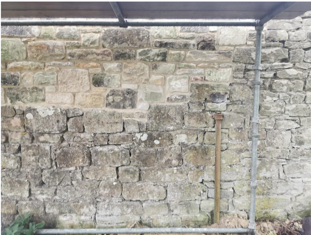
Photograph No. 2 – typical condition of masonry
