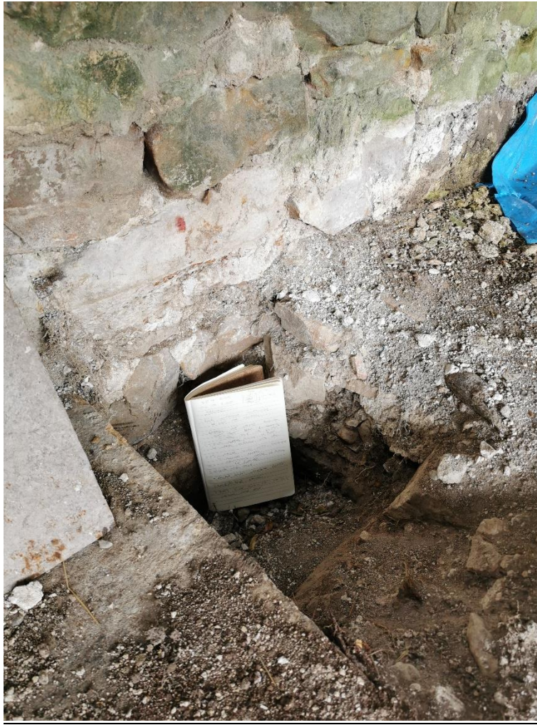
Photograph No.7 – trial pit indicating base of wall
