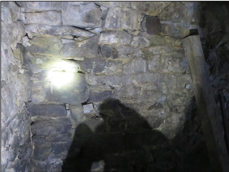
*Figure 49. Numerous gaps and crevices within ground floor walls.*
