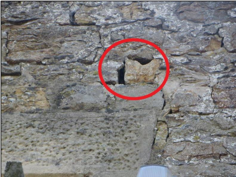
Figure 27. Close of up gaps present on the gable end wall of the granary.
