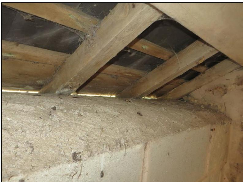
*Figure 63. Wall tops sealed on front elevation of cart shed.*
