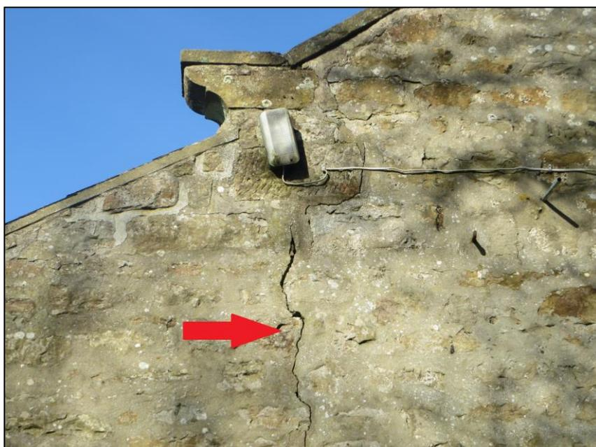
*Figure 14. Cottage – gable end wall crack present.*
