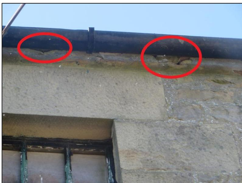
*Figure 31. Gaps present at wall tops above the window where bat droppings were found internally.*
