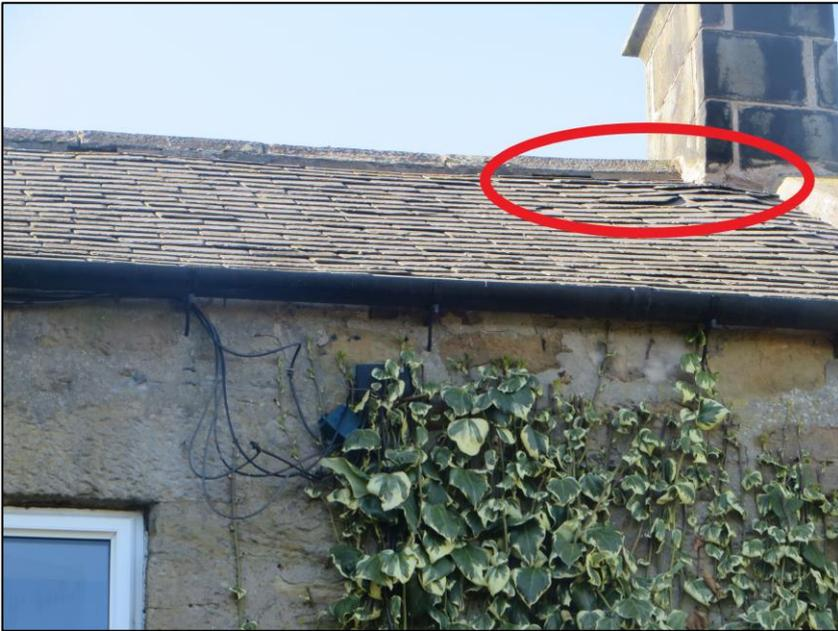
Figure 21. Misaligned tiles on farmhouse roof.
