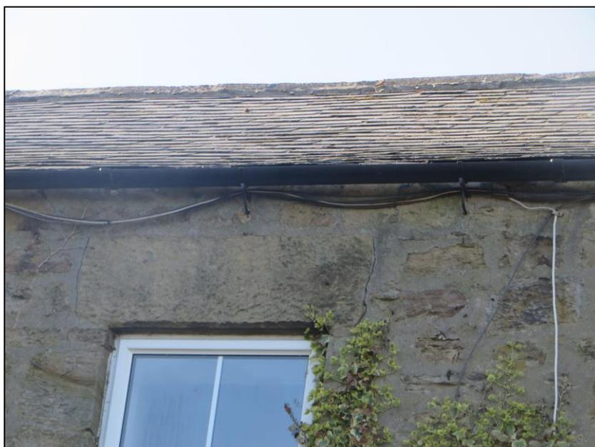
*Figure 20. Farmhouse roofline in regions where gaps were seen at wall tops.*
