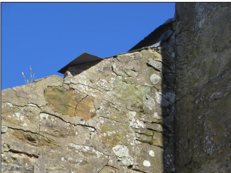
*Figure 53. Lifted lead flashing on cart shed roof.*
