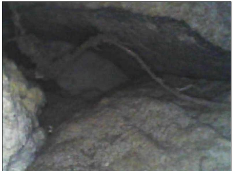
*Figure 58. Endoscope image of a cavity within the stone walls of the cart shed.*
