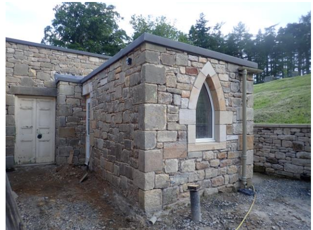
The garden room from the southeast
