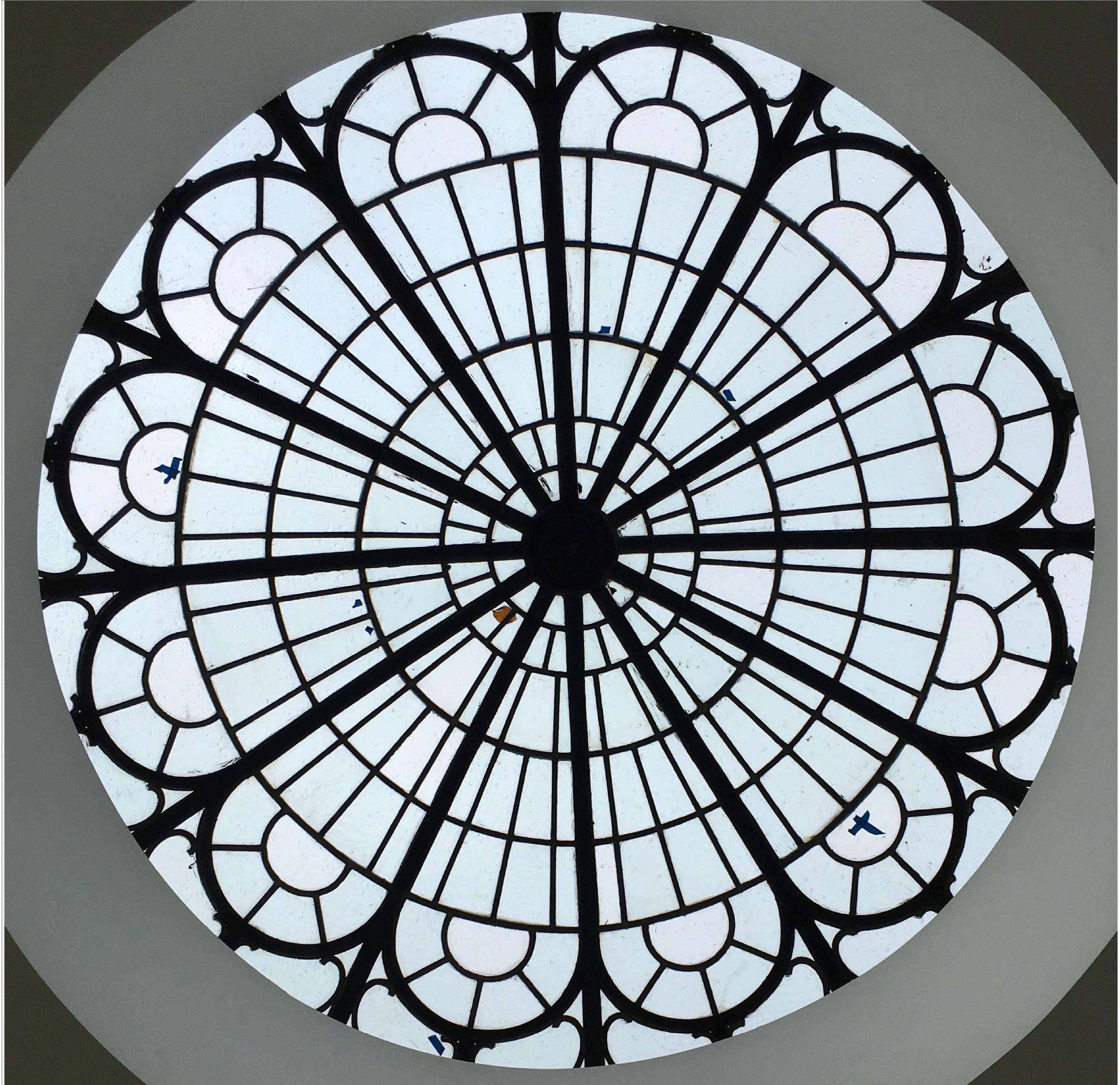
DOMES INTERNAL VIEW
