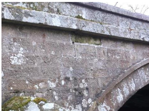
Photograph 6 Examples of failing brick-work and crevices in bridge.
