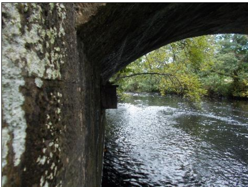
Image 4: Dipper box beneath bridge arch
