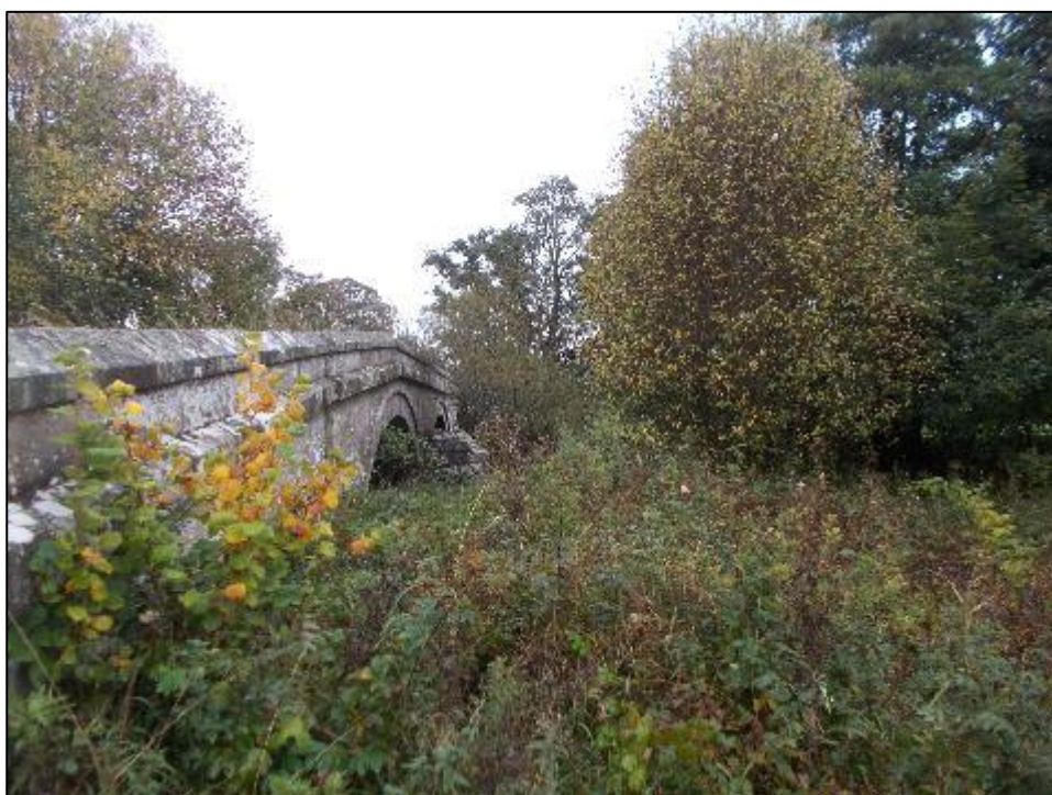
Image 2: Bridge north-west side with tall ruderal vegetation
