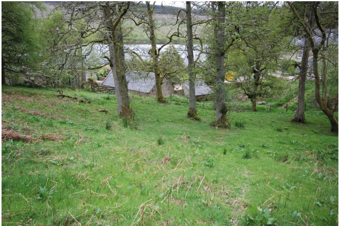
PHOTO 008 NORTH & EAST ELEVATIONS – FROM HILLSIDE ABOVE
