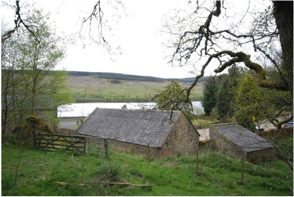
PHOTO 007 NORTH & EAST ELEVATIONS – A68 & RESERVOIR BEYOND
