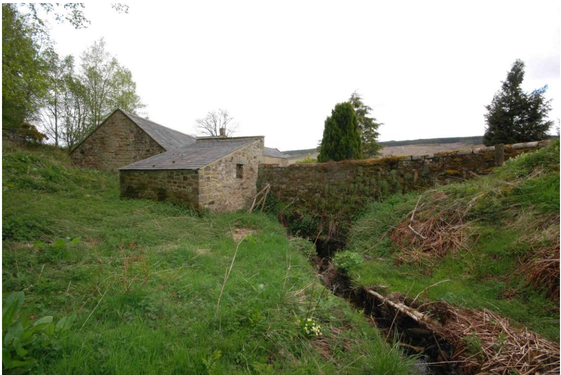
PHOTO 006 NORTH ELEVATION AND STREAM
