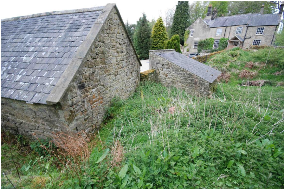
PHOTO 004 NORTH & EAST ELEVATIONS - CATCLEUGH FARMHOUSE BEYOND
