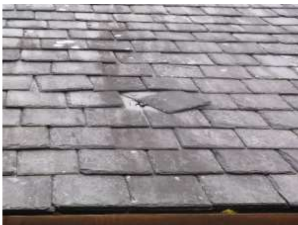
Photograph 5 – Example of loose roof slates
