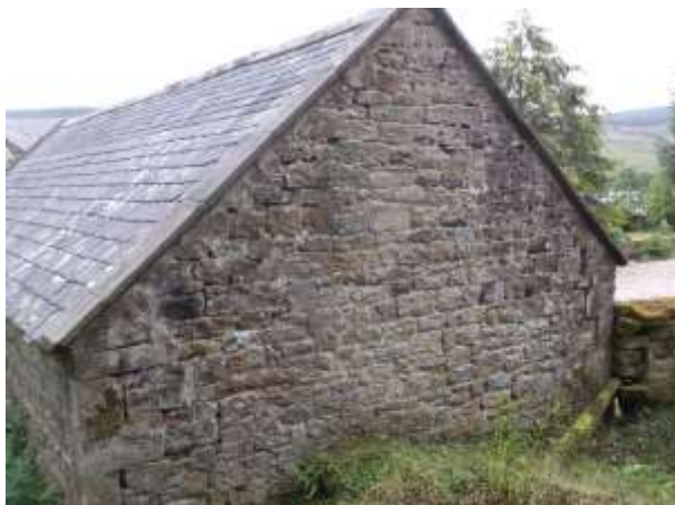
Photograph 5 – Example of loose roof slates
