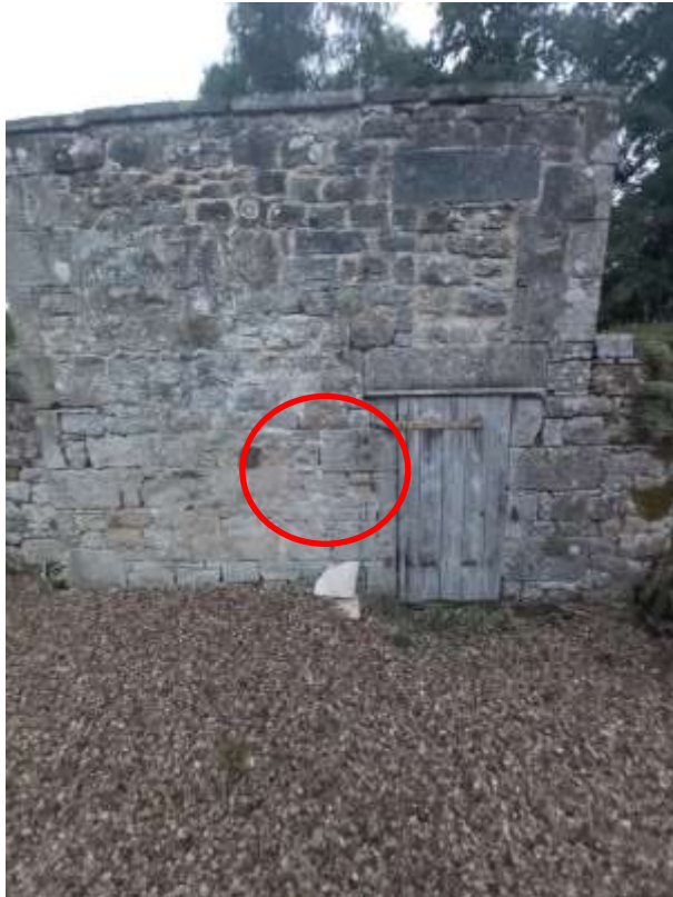
Photograph 11 – Location of roost within wall of stone storage shed.
