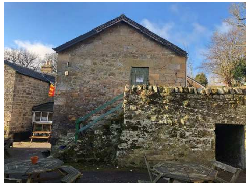
View of existing steps from Courtyard
