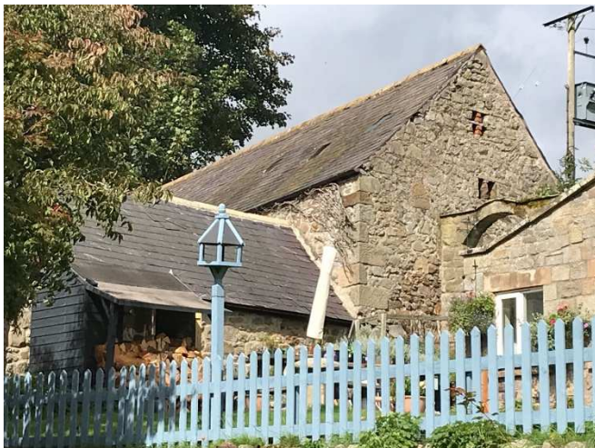
View of Buildings from East on Main Street
