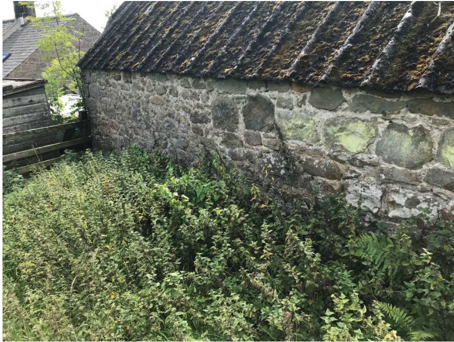
P3 – Asbestos cement roof sheets to north roof slope
