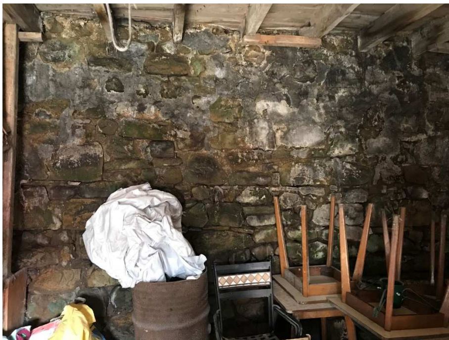
P4 – View of interior of former stables
