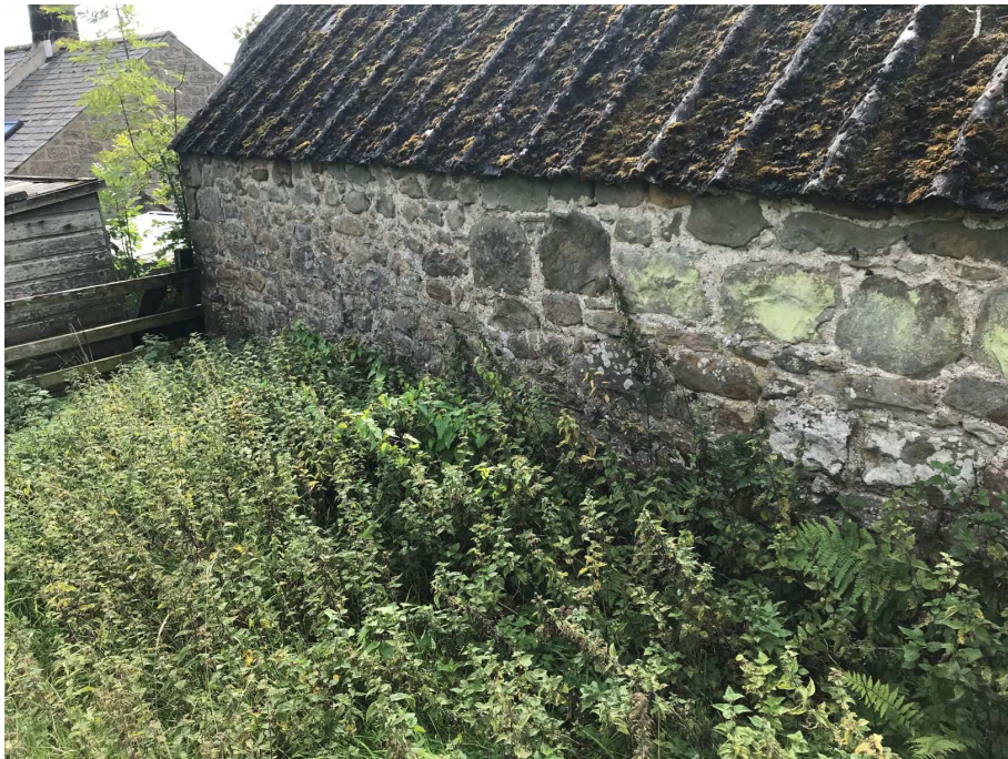
P3 – High ground level at rear of two-storey building
