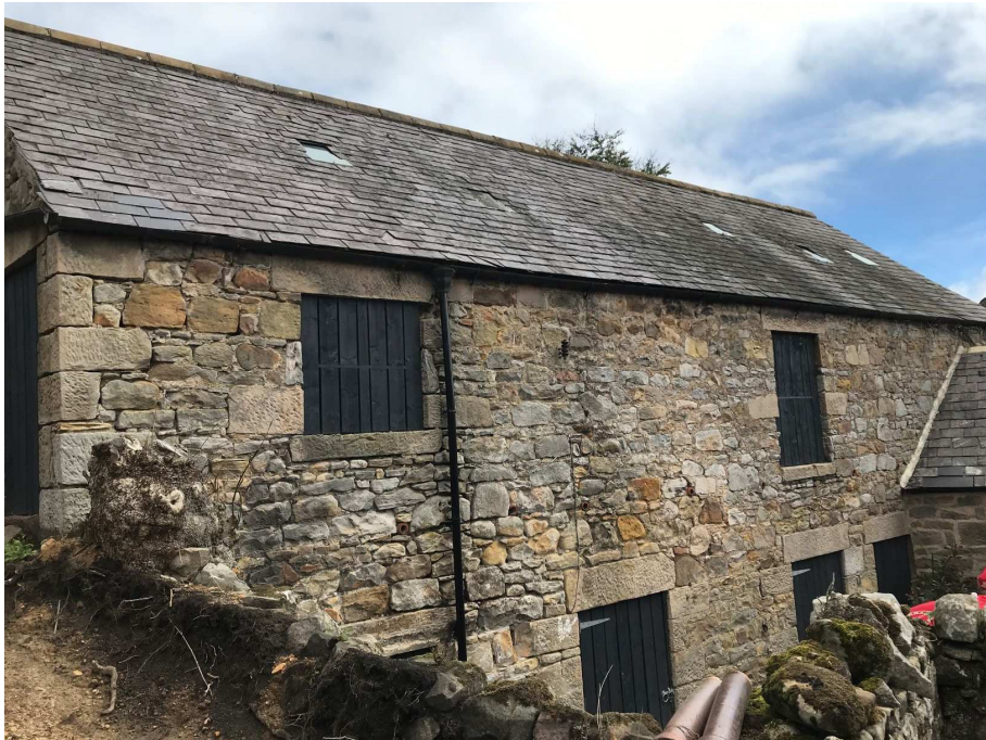
P1 – View of two-storey building
