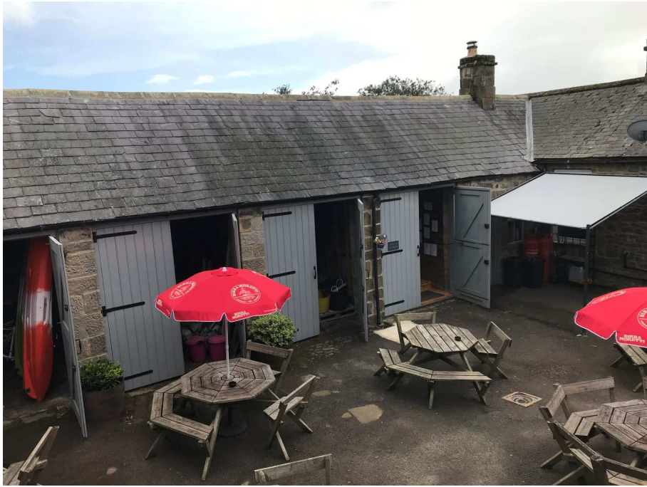
P9 – View of single-storey garages / roof coverings
