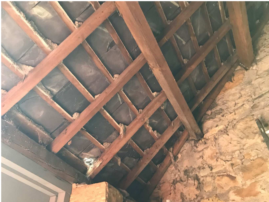
P14 – View of garage walls / roof structure
