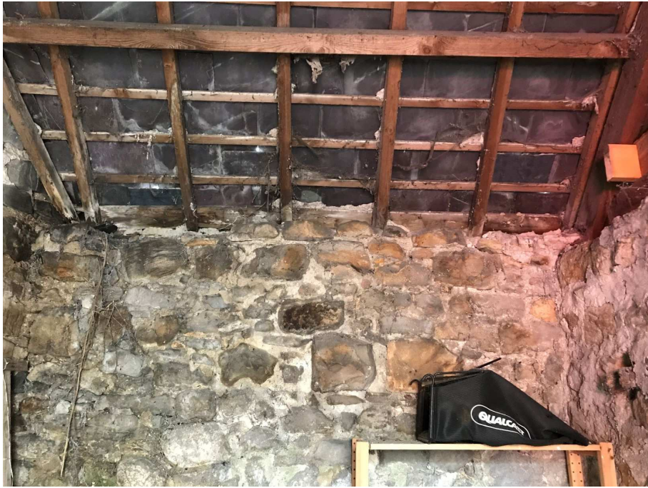
P13 – View of garage walls / roof structure
