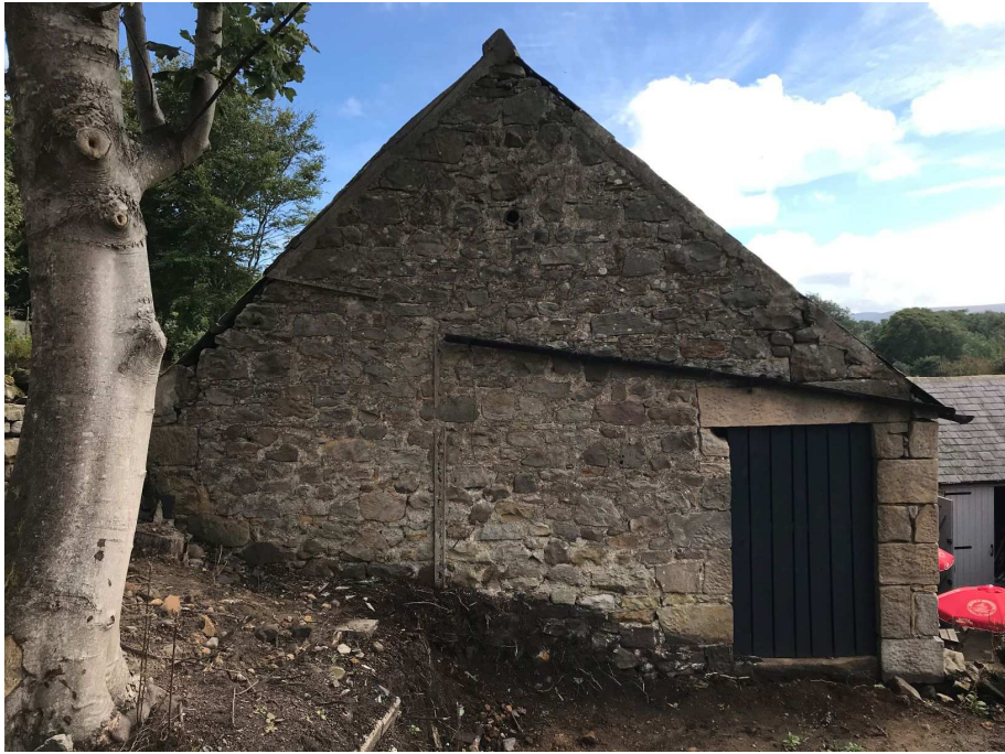
P5 – West gable wall
