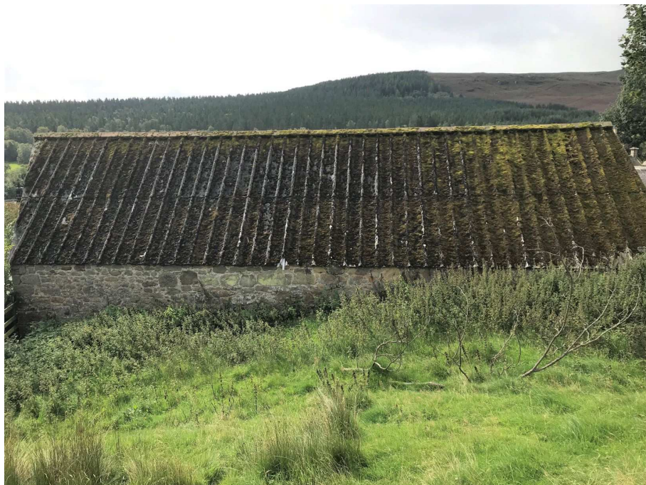
P2 – Rear of two-storey building / asbestos roof sheets
