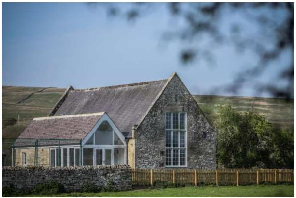
The side extension to Greystead Institute was added during its conversion in 2018. The Garden Room (below) reflects the existing building, with a slate roof, stone walls, and timber windows and doors. It is located on the western elevation in the location of a previous lean-to extension, and is set back from the north 'frontage' gable wall.
