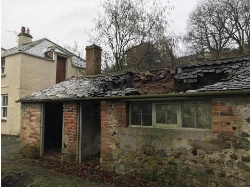
Figure 2: Previous outbuilding located within the footprint of the proposed building
