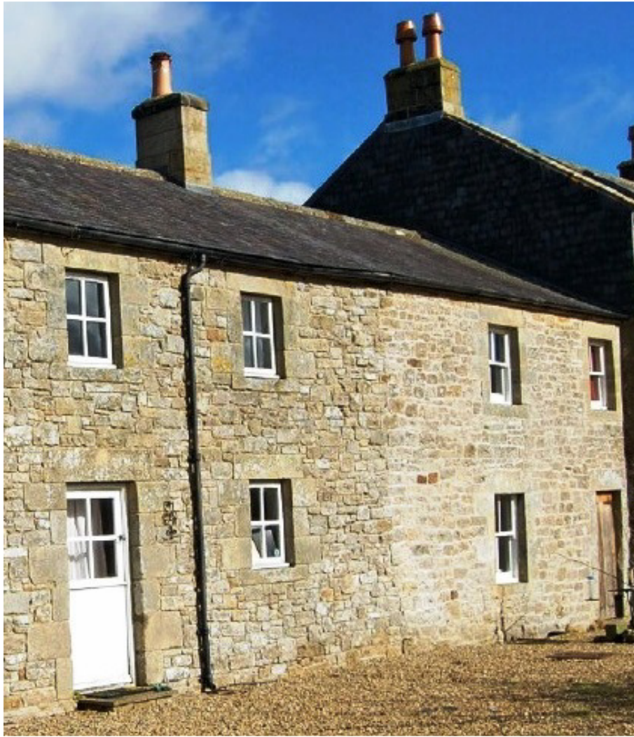
Existing Kitchen stable door
