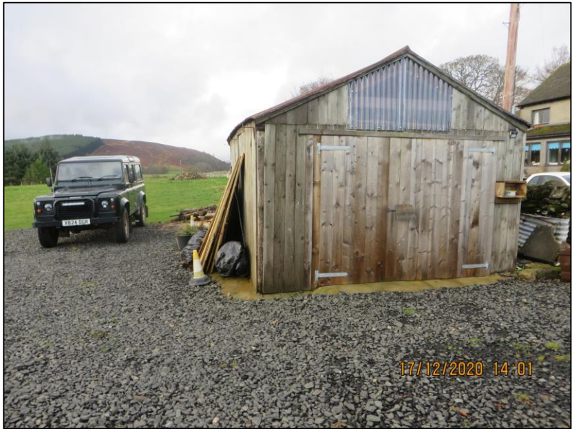
Figure 15. Shed by site entrance.
