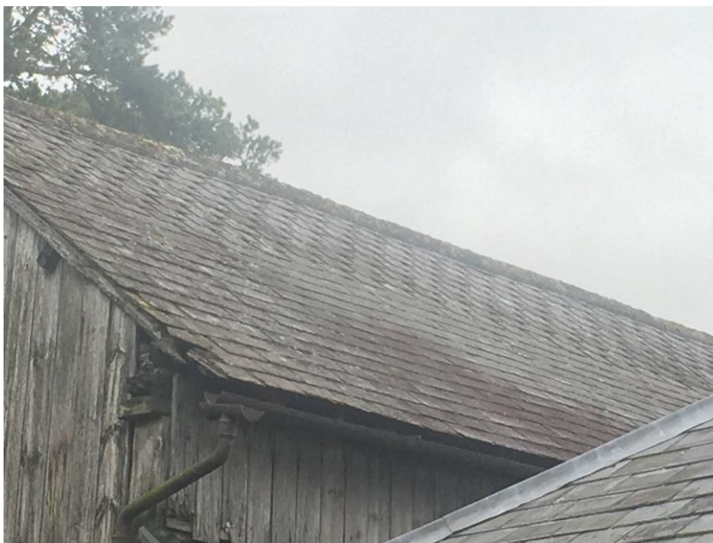
Photograph 10: Exterior of roof of wooden barn
