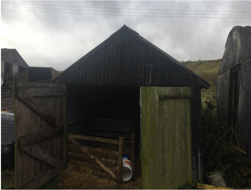
Photograph 1: Corrugated metal shed
