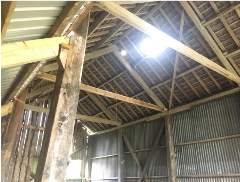
Photograph 9: Interior roof of wooden barn
