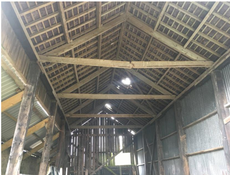
Photograph 8: Interior roof of wooden barn
