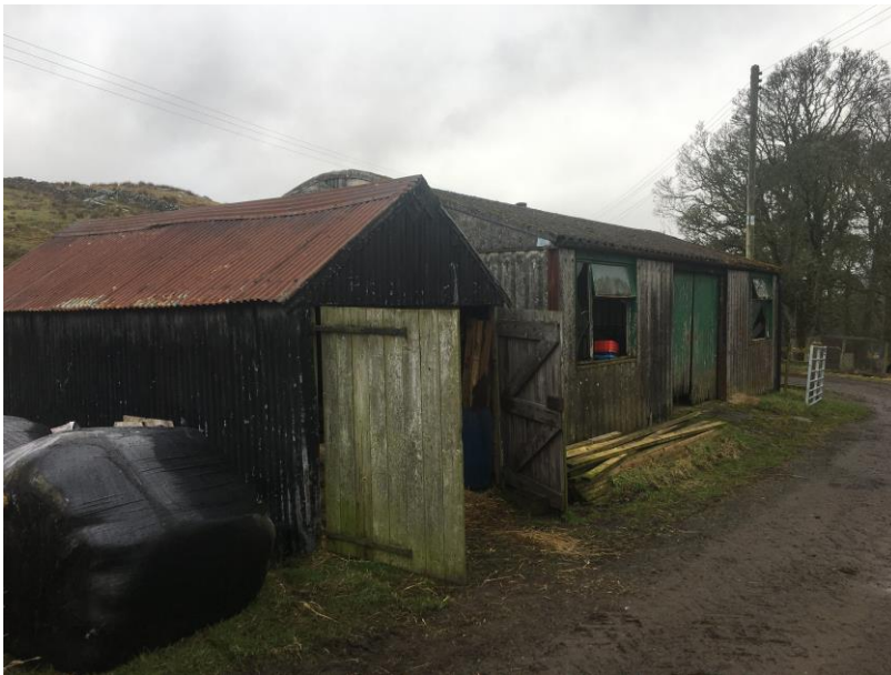
Photograph 2: Corrugated metal shed with asbestos shed behind
