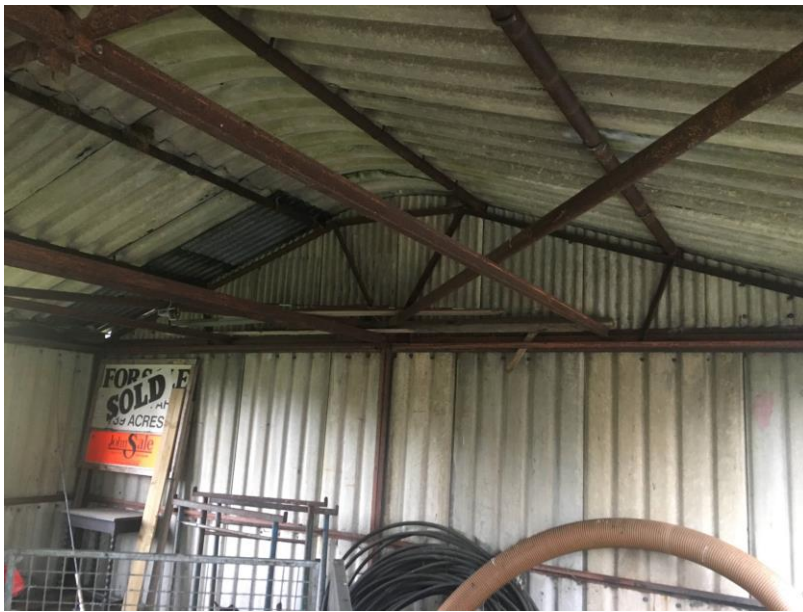
Photograph 4: Interior of asbestos shed
