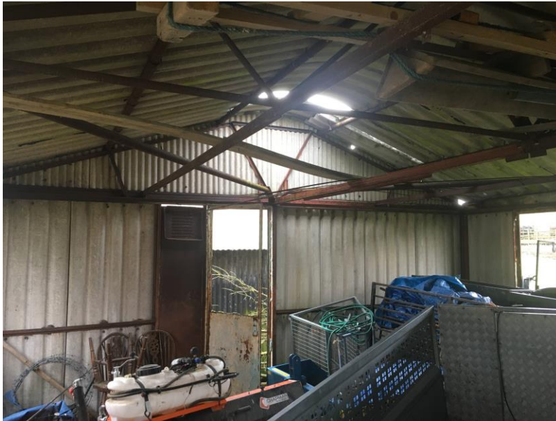
Photograph 5: Interior of asbestos shed
