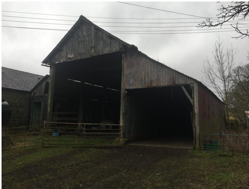
Photograph 12: Separate garage on right that is part of wooden barn
