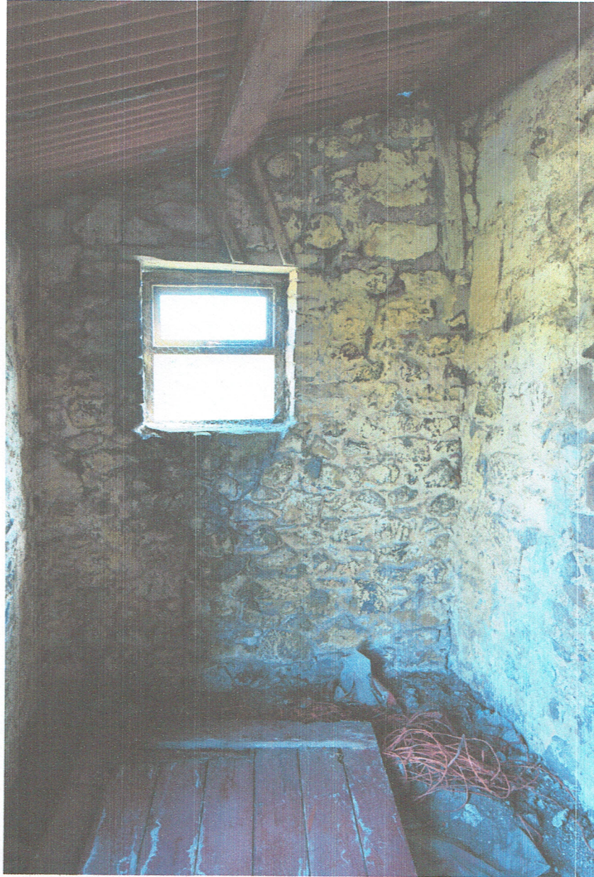
Photograph D (Lean-to)
