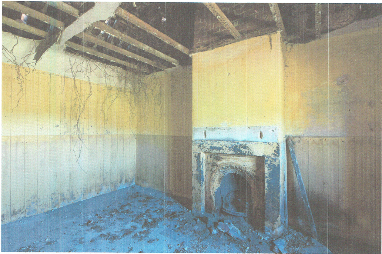
Photograph A (Bedroom)
