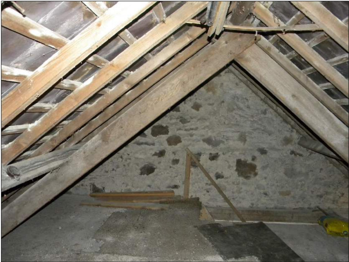
Figure 27. Building C. loft
