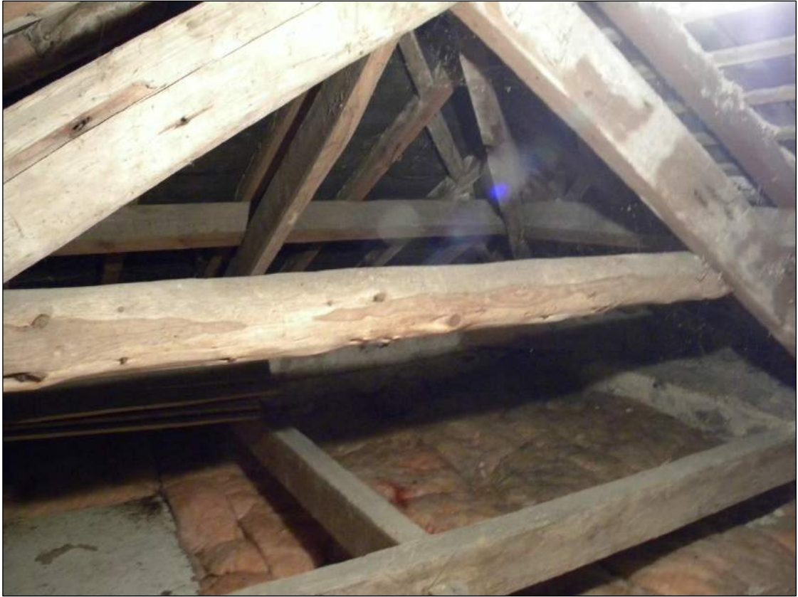
Figure 9. View of the loft
