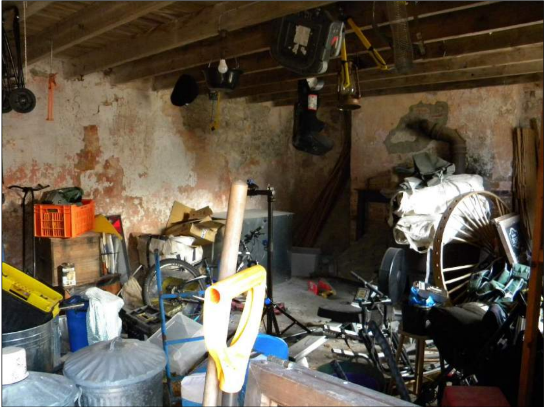
Figure 29. Building C. lower floor of outbuilding (eastern section).
