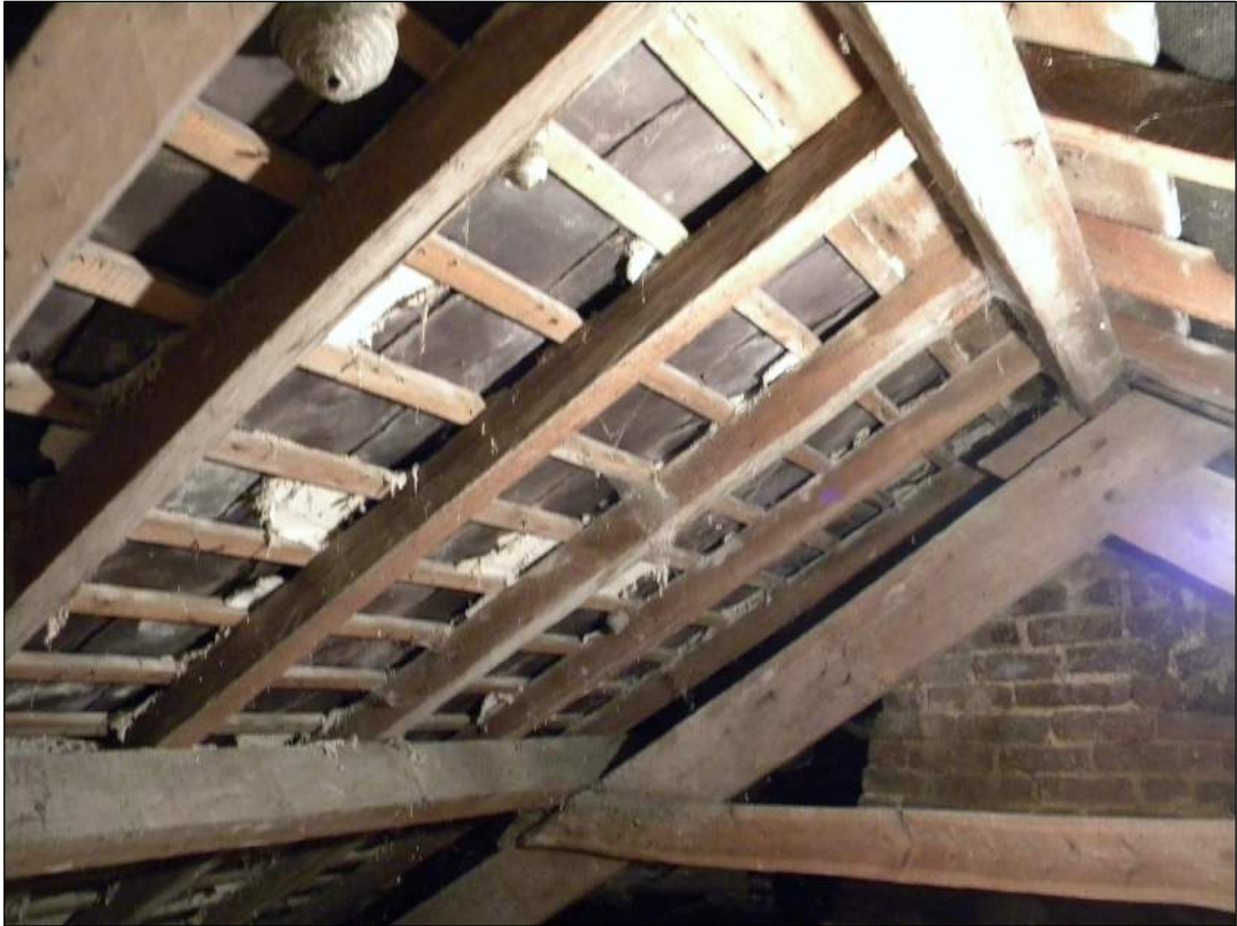
Figure 11. Bare slate to underside of north elevation pitched roof of farmhouse.
