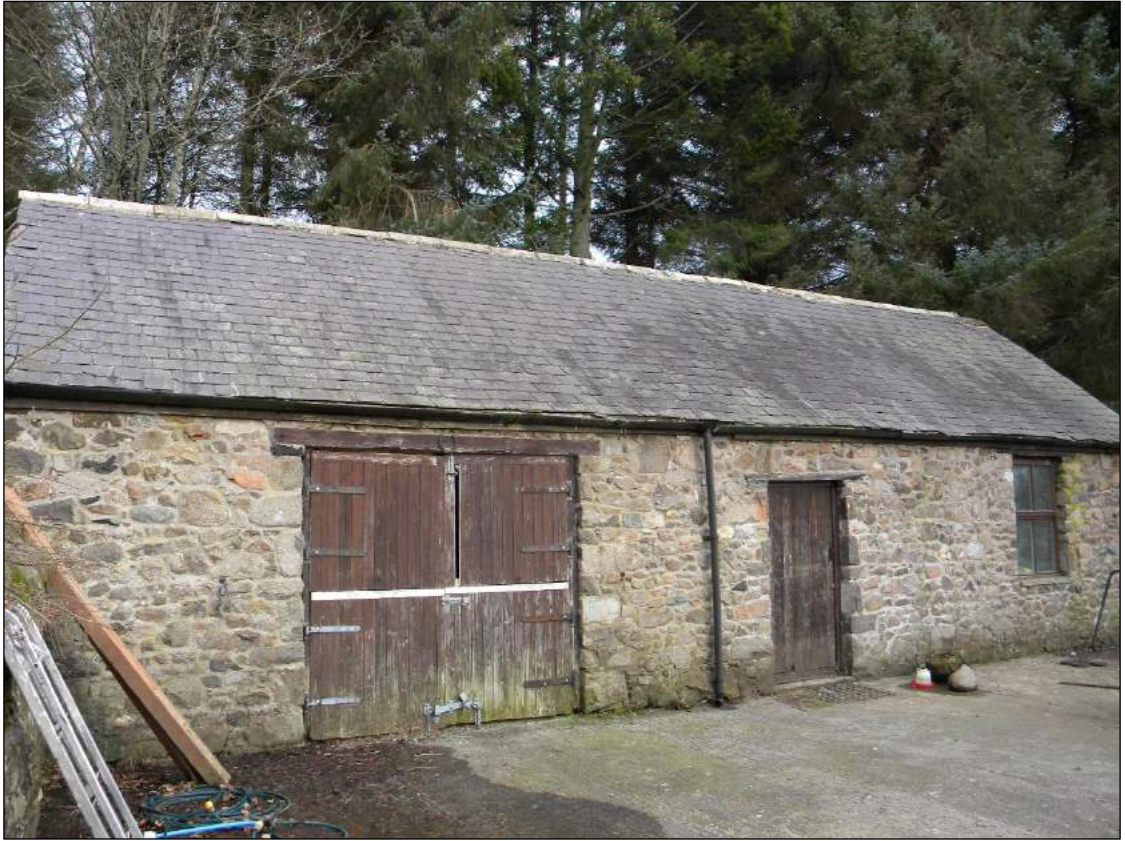
Figure 25. Building C. outbuilding
