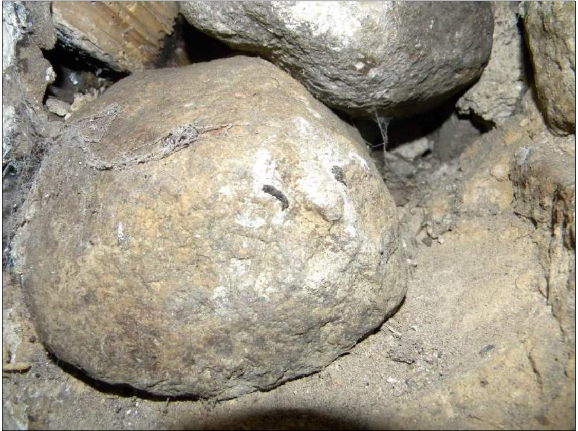
Figure 22. bat dropping to the wall of the stables.
