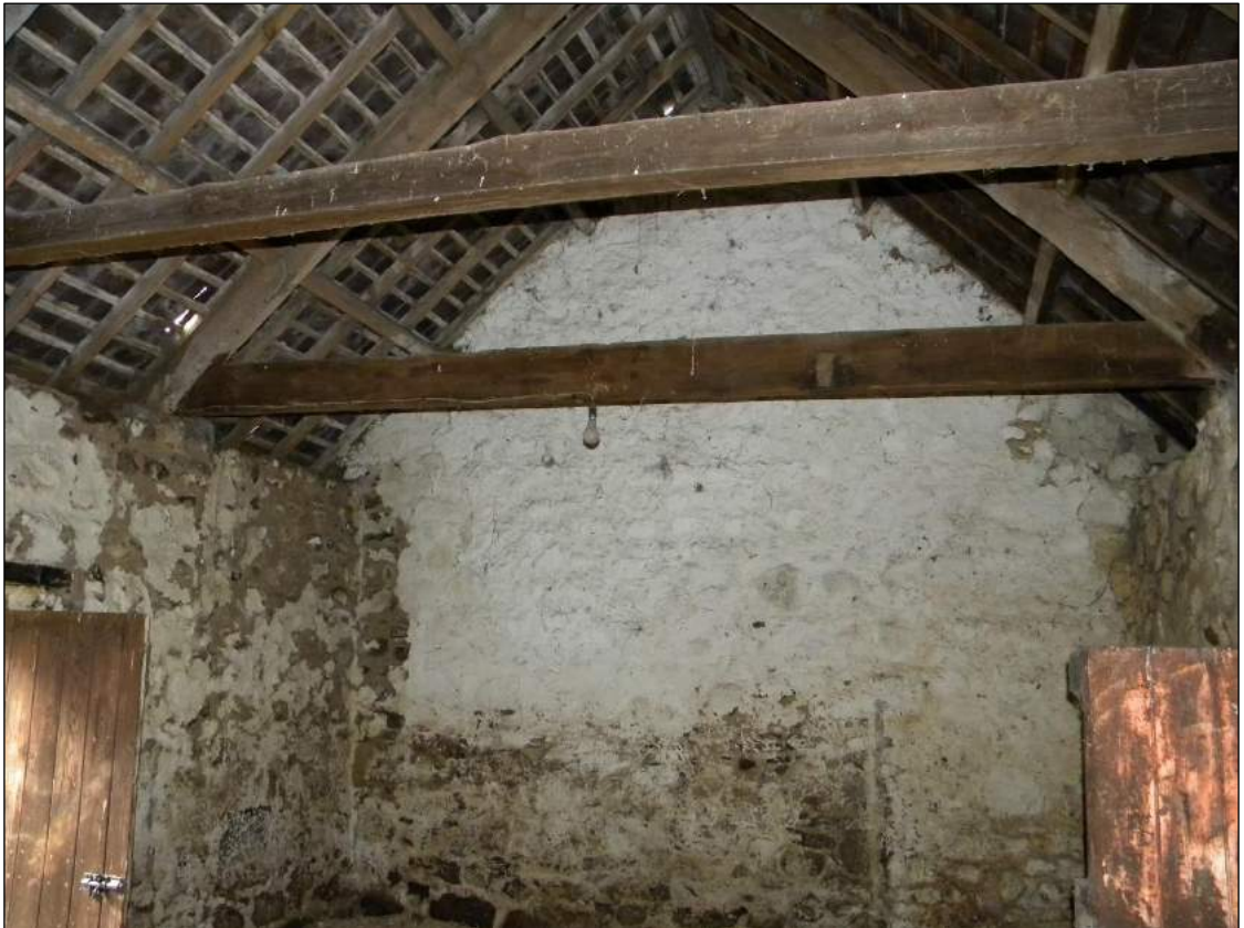
Figure 21. Interior of stables, eastern side showing unlined roof .
