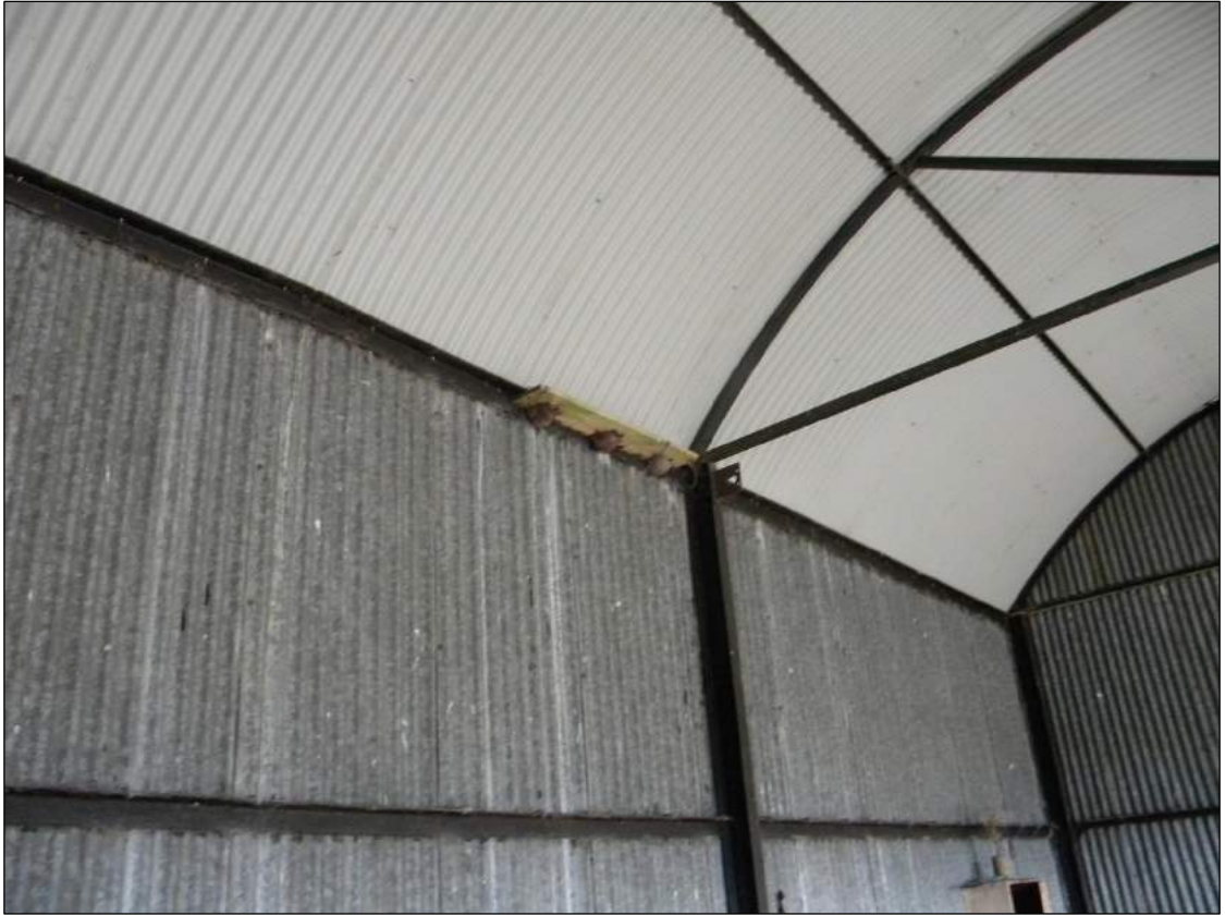
Figure 31. Building D. Swallow nest cups in steel barn.
