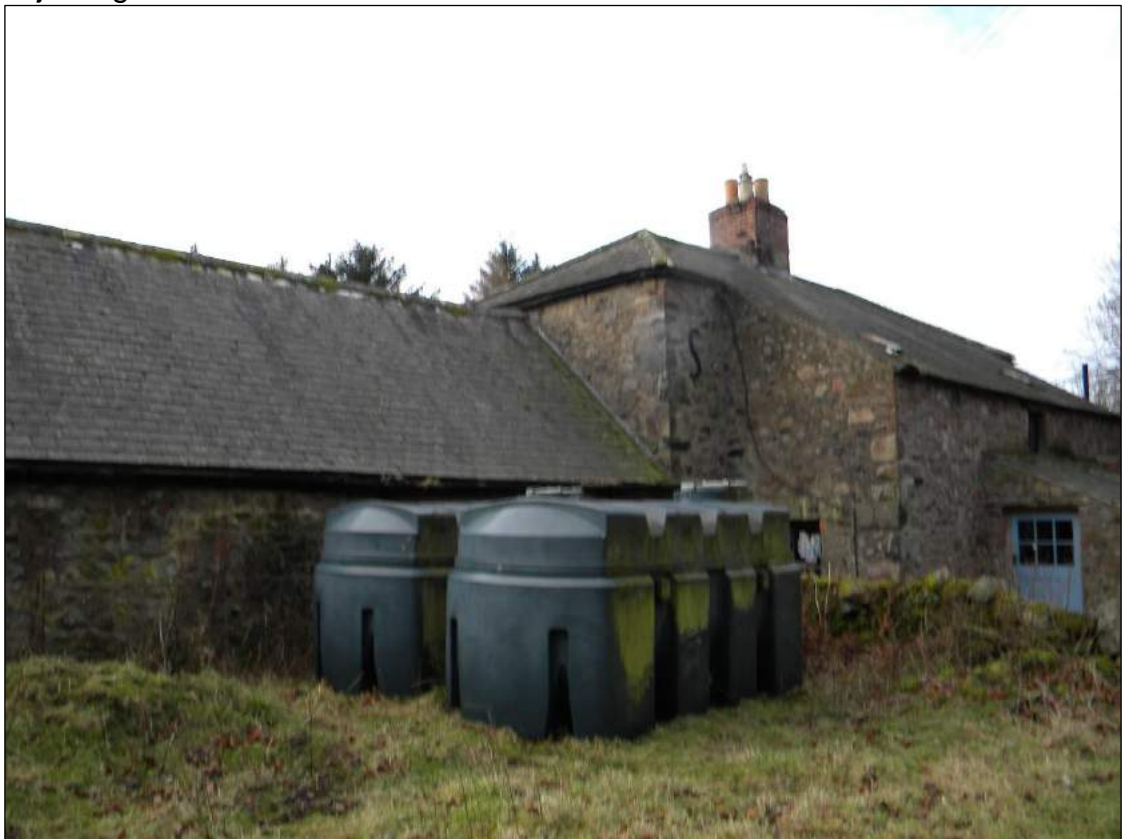
Figure 19. north elevation of building B – stables adjoining farmhouse.
