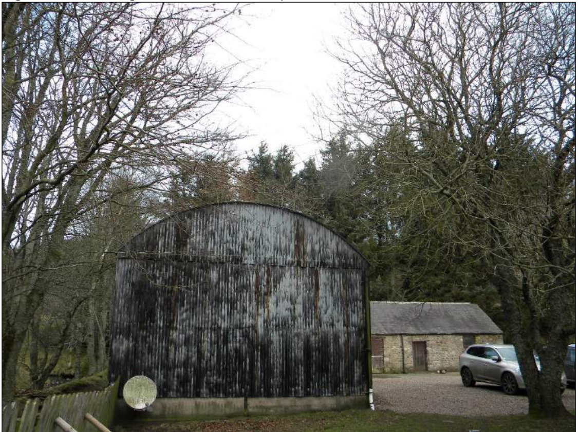
Figure 32. Building D. Steel framed metal sheeting Dutch Barn.
