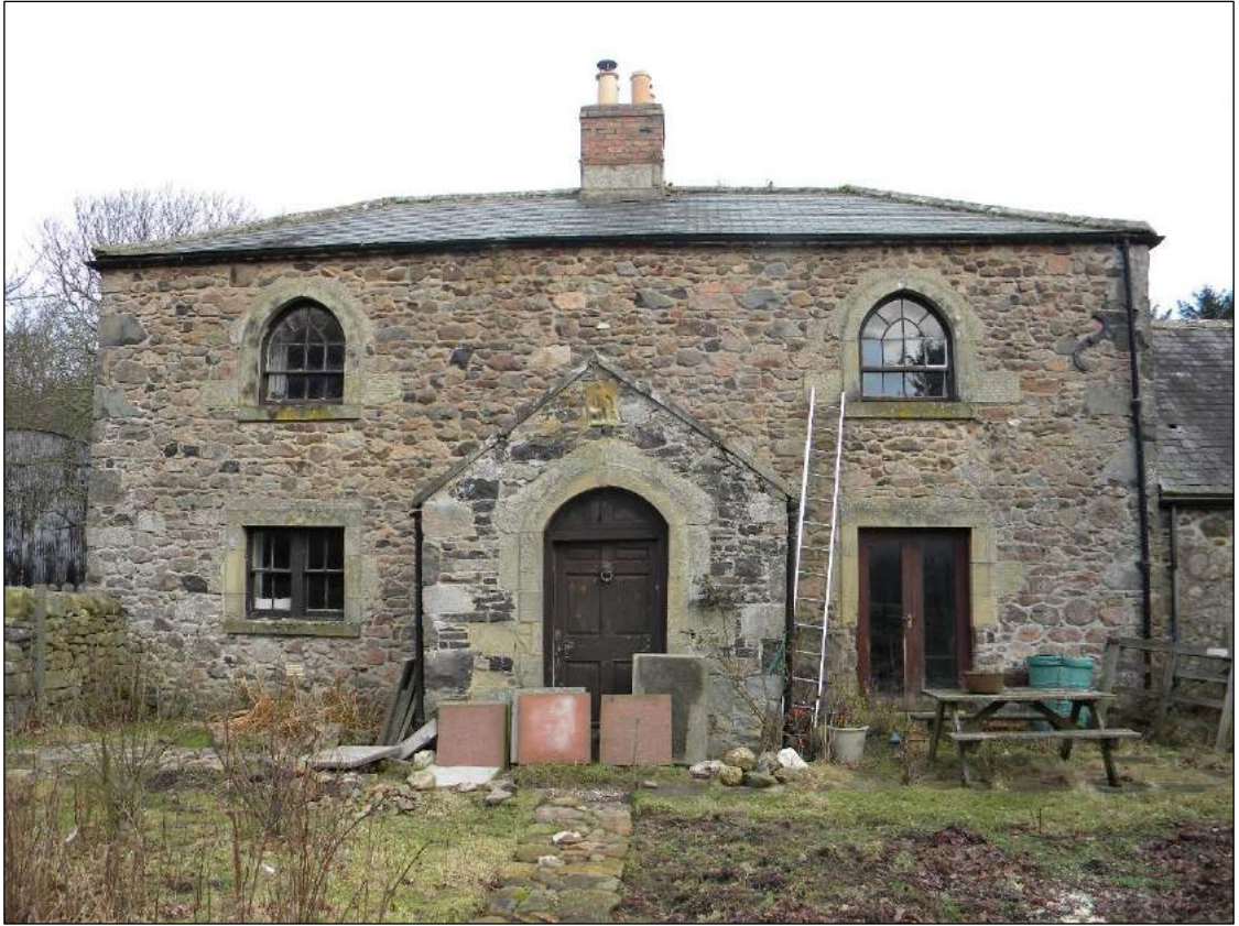
Figure 17. South elevation of farmhouse.
