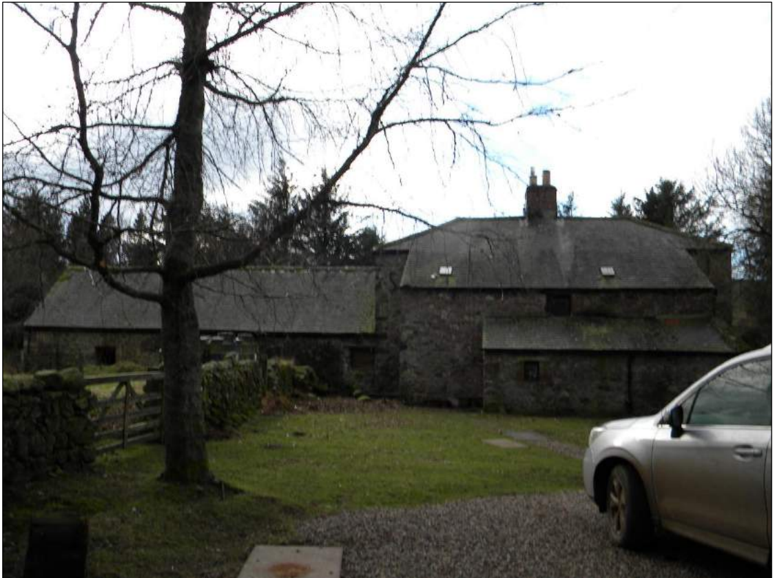
Figure 16. north elevation of farm house .
