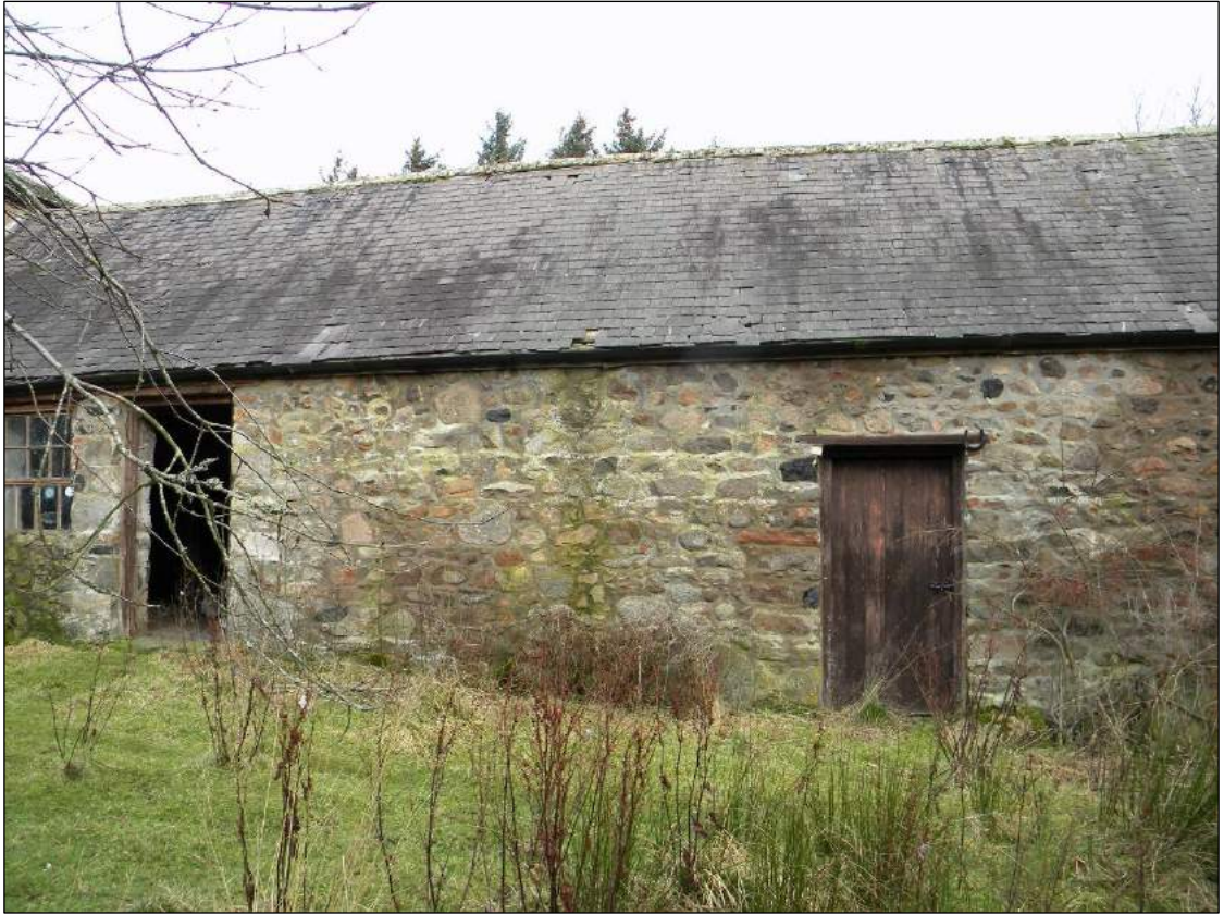
Figure 20. south elevation of building B – stables adjoining farmhouse.
