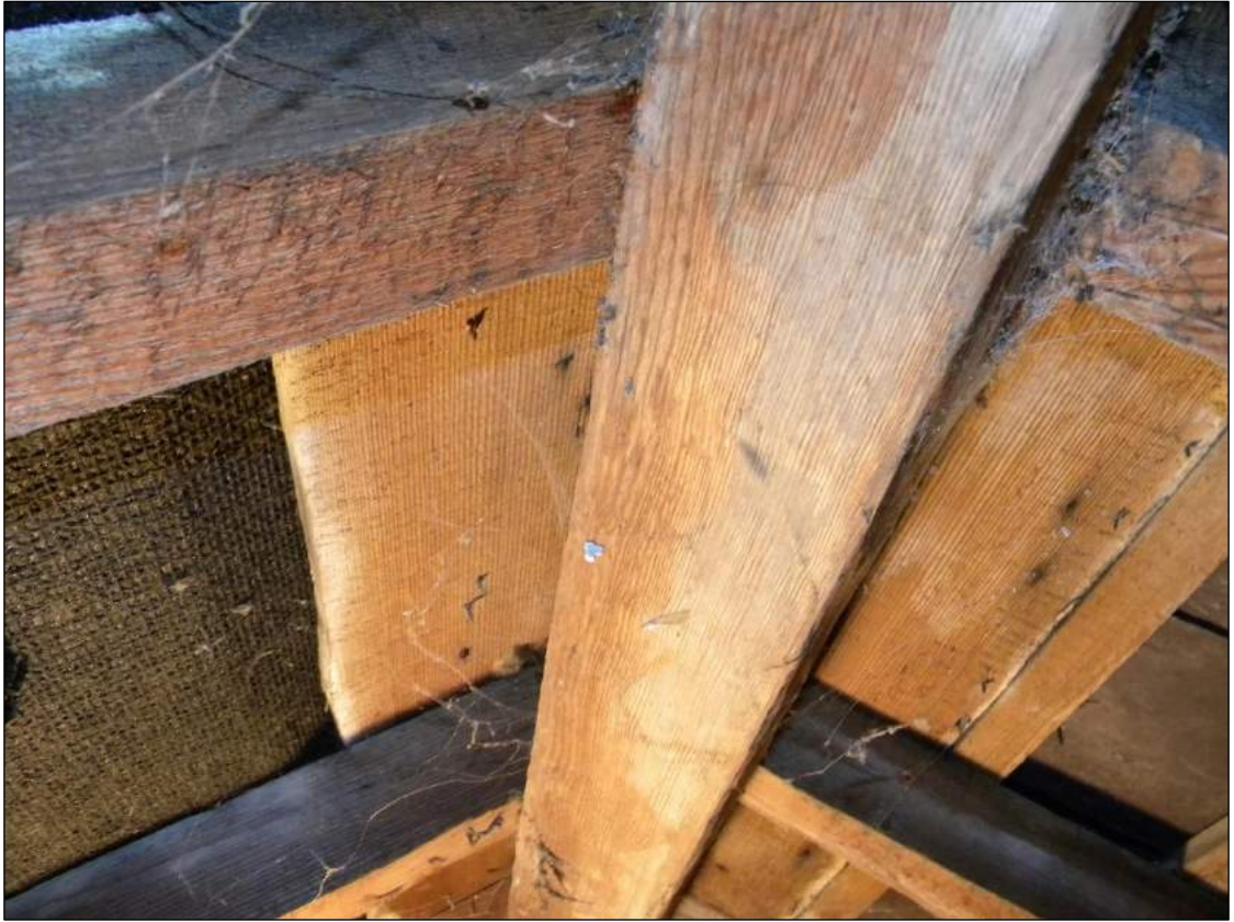
Figure 13. Timber to underside of ridge.
