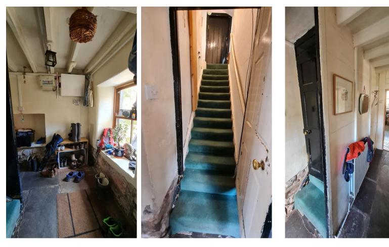
The current stairs are enclosed and run against the side of the original building. They are in a dreadful state with woodworm and rot – literally being held together with carpet!
