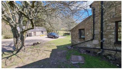
This elevation shows the large window that was unsympathetically installed in the 70s. The window leaks badly when it rains. Builders have said that if we don't deal with it, the wall will bow. To the left of the large window on the 1<sup>st</sup> floor we intend to install another window for the amended room configuration.
