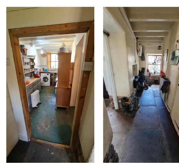
There is a temporary kitchen in here currently. The left hand side of this whole area is the side of the original building and we will strip this back to bear stone, as behind the plasterboard is constant habitat for rodents. We will install a new kitchen and floor as well as moving the Aga / Cooker in.
