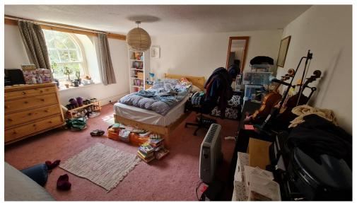
A lot of remodelling is required in this room. A ceiling has been installed in this room that is both too low and cuts off the top of the gothic shaped window inlet. It needs taking down and replacing.
