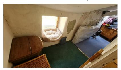
The aforementioned corridor configuration is bad space that is created by the badly sighted stairs. Some of the exterior walls are damp and will be exposed to understand the issues. Likely the badly fitted skylights and overflow from guttering. The skylight will be replaced with Heritage equivalent and provide light over the new stairs
