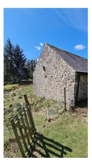
The gable end adjacent to the river. The soil will be brought down to expose the original ground level to avoid issue with damp later.
