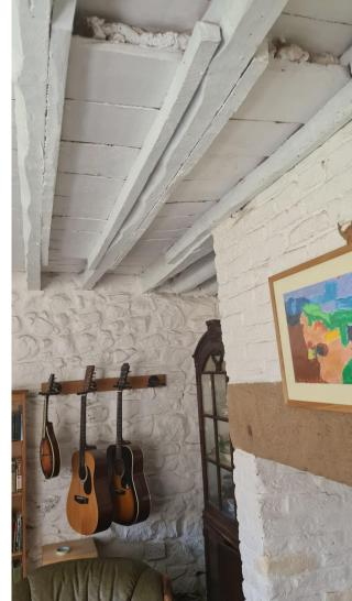
There are a number of areas that need addressing in this room. The large unsympathetic (and leaking!) window will be reduced in size so that it no longer threatens the structural integrity of the wall.
