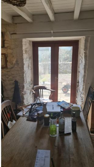
There are a number of areas that need addressing in this room. The patio doors will be reinstated as a window. Between the Piano and the freezer there will be a new doorway to provide access to barn 1. The Aga will be uninstalled and a new stove fitted
