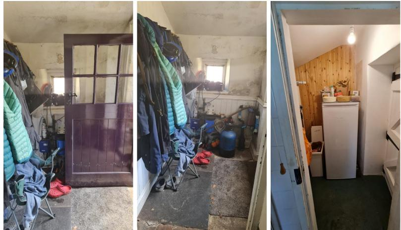
The tongue and groove partition with the coats on will be removed to open up into a new utility room. The other side of the tongue and groove has the freezer in front. There is no wall just the wood loosely fitted to the gap.
