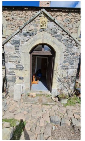
The barns adjoin our current house. Here we can see the patio door that we wish to re-instate as a window and the porch that will need to be rebuilt to make it weather proof using existing materials.
