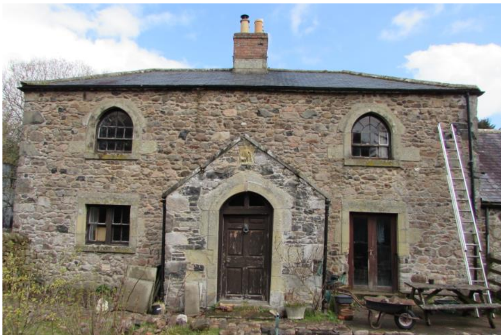
Figure 3: Southern elevation showing porch to be rebuilt.
