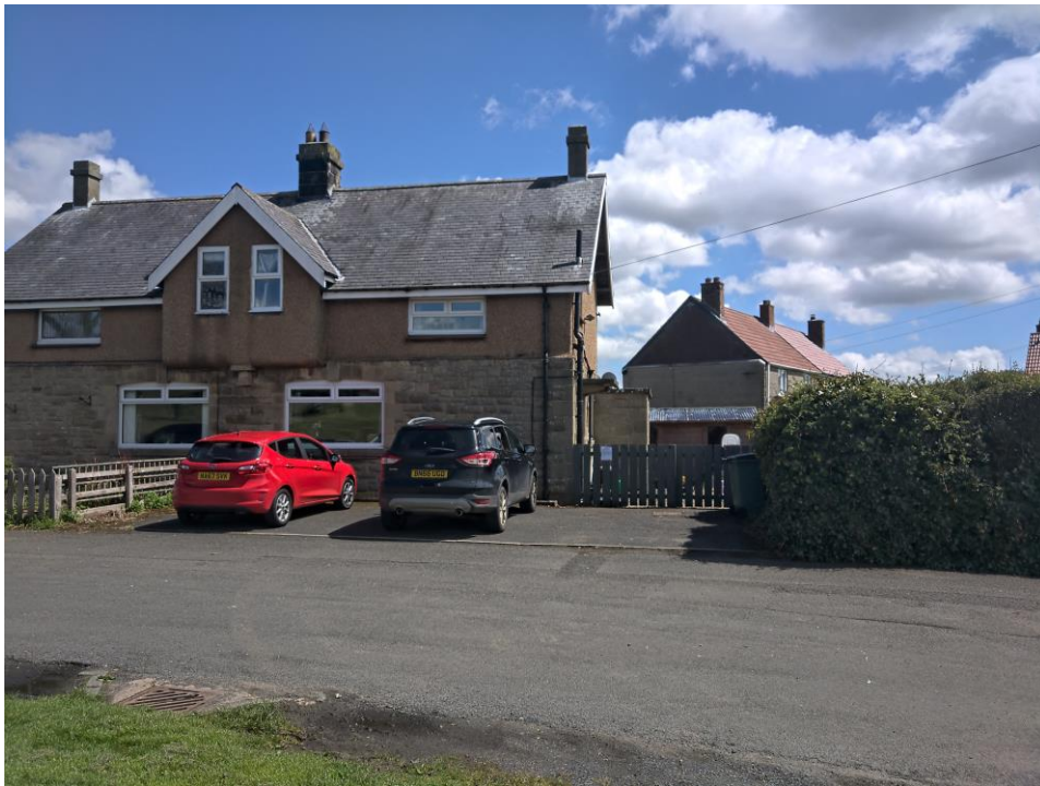
Figure 3: Application site highlighting existing materials.
