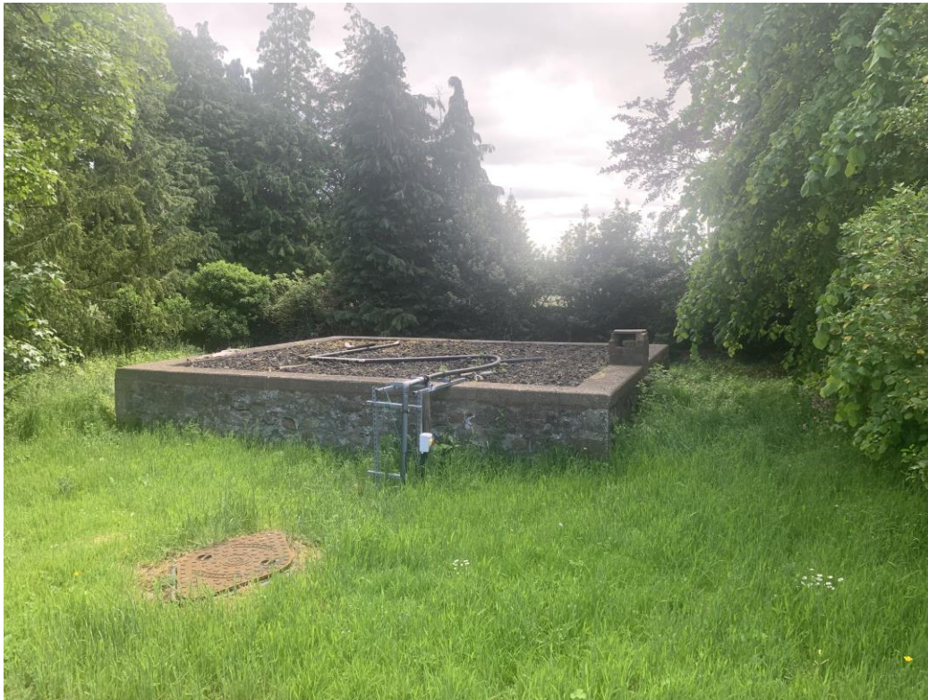
Figure 2: Septic Tank currently in place at Yearle House
